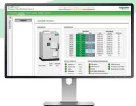
Remote power factor monitoring center
